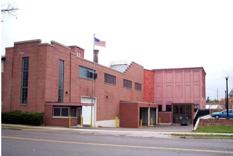
The Gibson building, an historic silk mill has had additions over the years that have not enhanced the character of the original structure.
