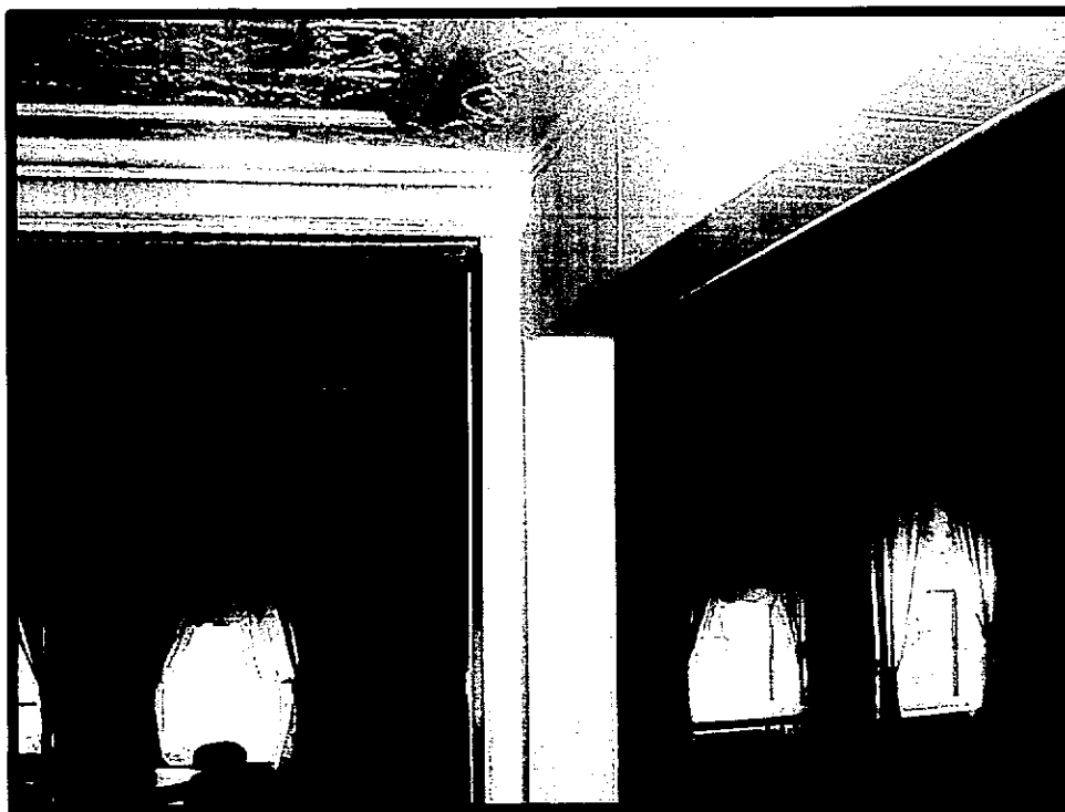
24. "LARGE HALL" LOOKING EAST. NOTE: PRESSED METAL CEILING TO THE LEFT AND POSSIBLE PLASTER OR DRYWALL CEILING TO THE RIGHT.
