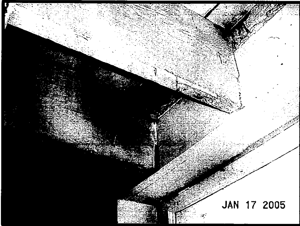
19. JOISTS BEARING INTO WOOD LINTEL AT BASEMENT WINDOW. NO JOIST HANGERS.
