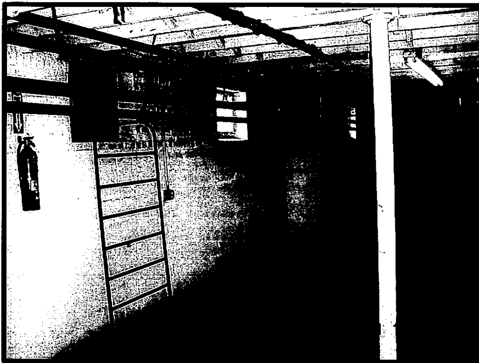
10. BASEMENT LOOKING N. EAST. NOTE: COLUMN SUPPORTS DOUBLE JOIST BELOW PARTITION LOCATION ABOVE.
